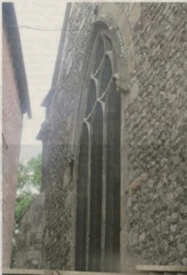
Work on the outside was completed on Wednesday of last week.
