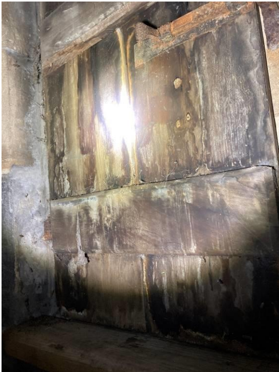
Access door to tower roof.
