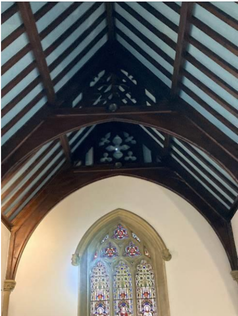
Nave roof structure
