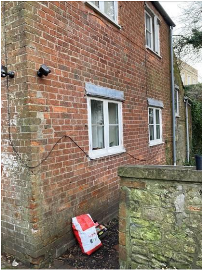
Curfew Cottage—south elevation
