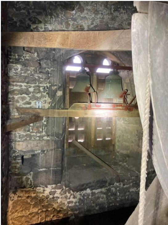
Quarter Jacks to north opening
