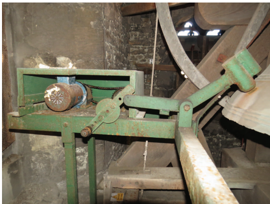
Electric curfew striking mechanism
