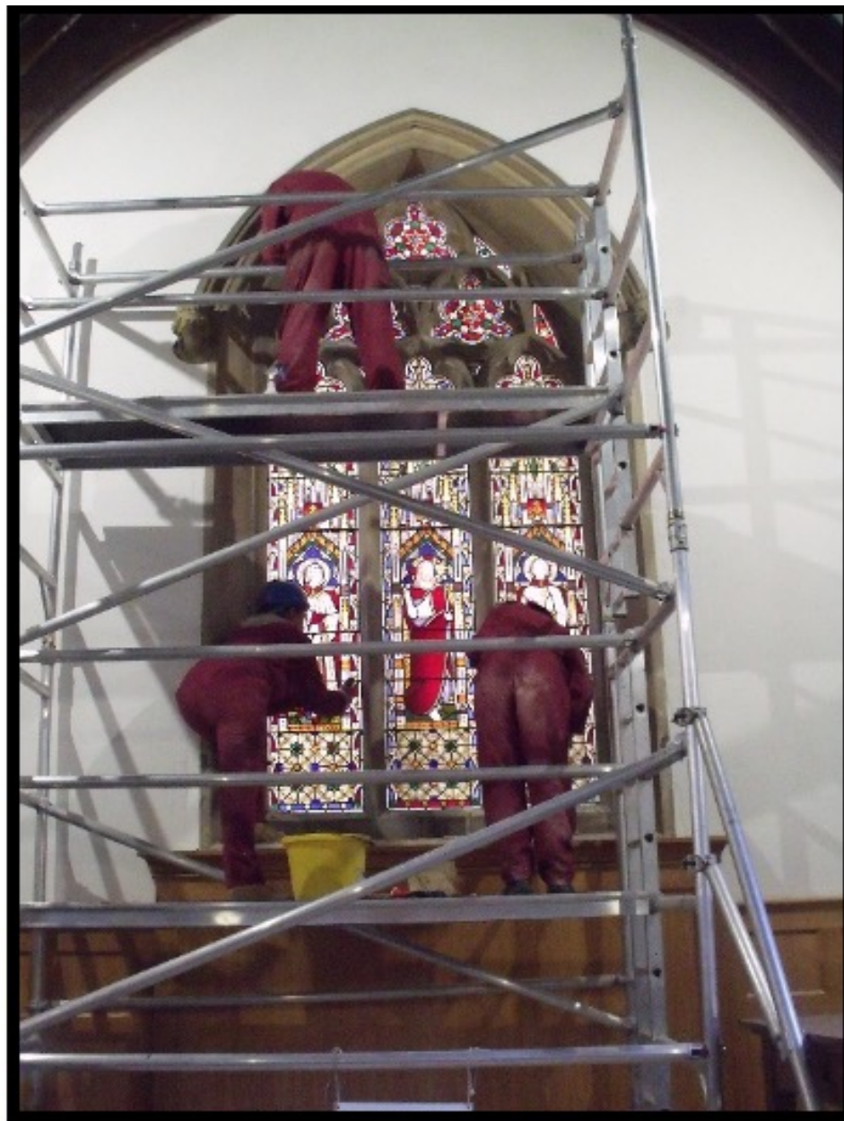
Finishing the internal fixing of the glazing
