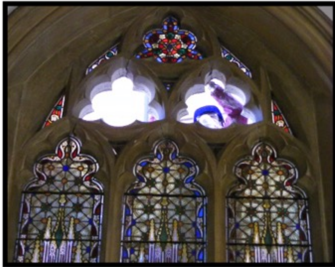
Removal of the glazing from the stonework
