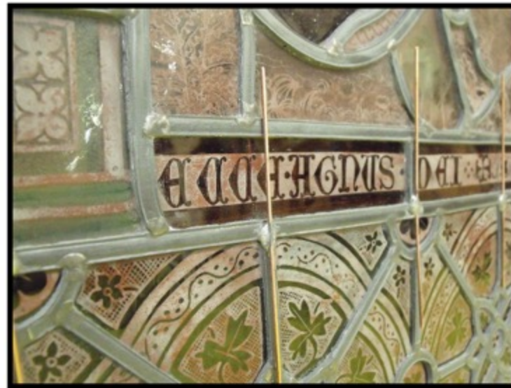
New copper ties solder to lead work joints
