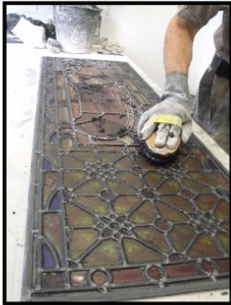
Re-leading on the original glass on the bench
