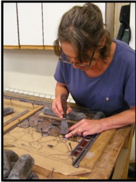
Re-leading on the original glass on the bench
