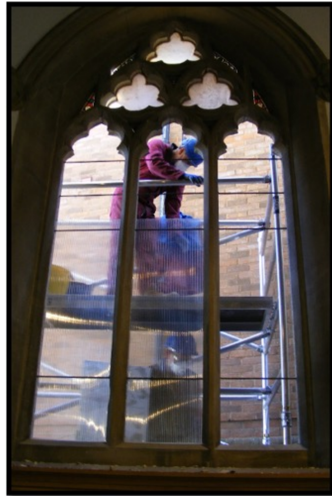
Removal of the glazing from the stonework
